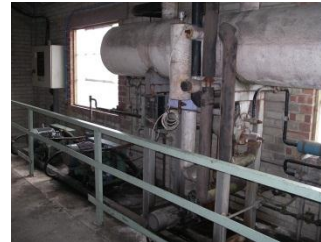
Fig. 2 Receiver and Witt Refrigerant Pump
