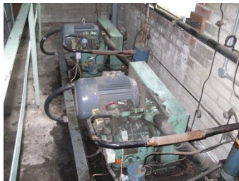
Fig. 1 Bitzer open drive reciprocating compressors
